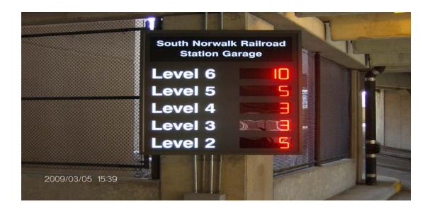
The installation of the parking level count system at the 720-space South Norwalk Train Station Garage was completed on March 5, 2009. The system allows staff to monitor space availability on a floor by floor basis. This information is provided to commuters as they enter through the upward helix.
